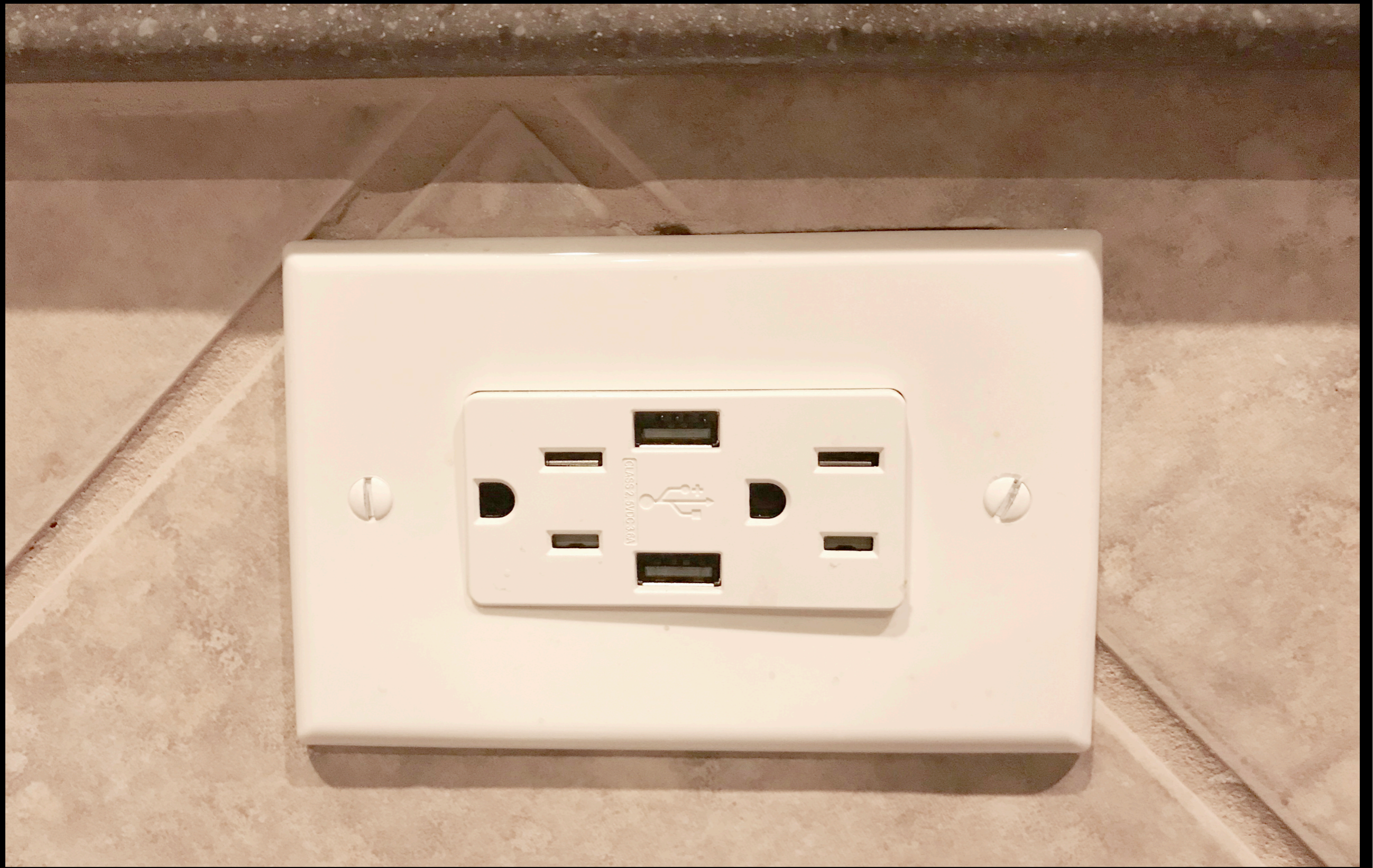
Wall Outlet with 2 USB Outlets
